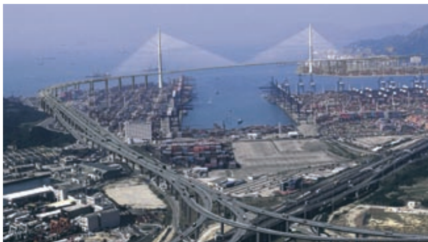
Outokumpu Stainless levererar stålet till Stonecutters Bridge i Hong Kong.
