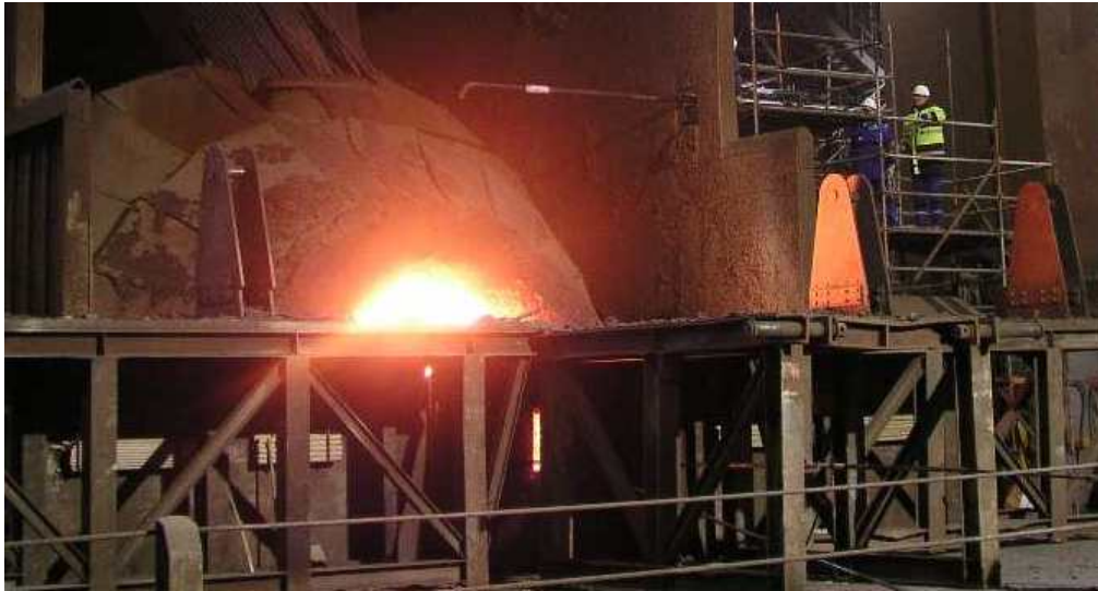
Figure 12 Installation of equipment for fume suppression
