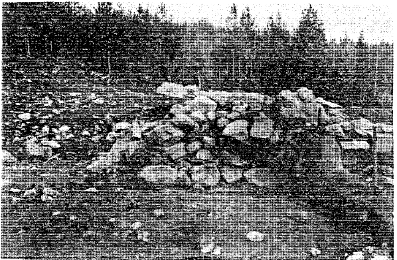
AI THE BLAST FURNACE, WESTERN WALL
