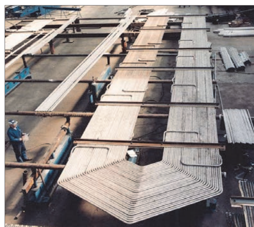
Figure 6.11.1 Manufacturing of super heater coil in steel Sanicro 25
